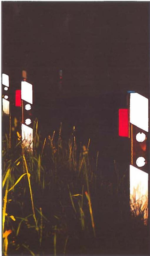
Immediately after the vehicle has passed, the reflectors become inactive, thereby permitting the animals to cross safely.
